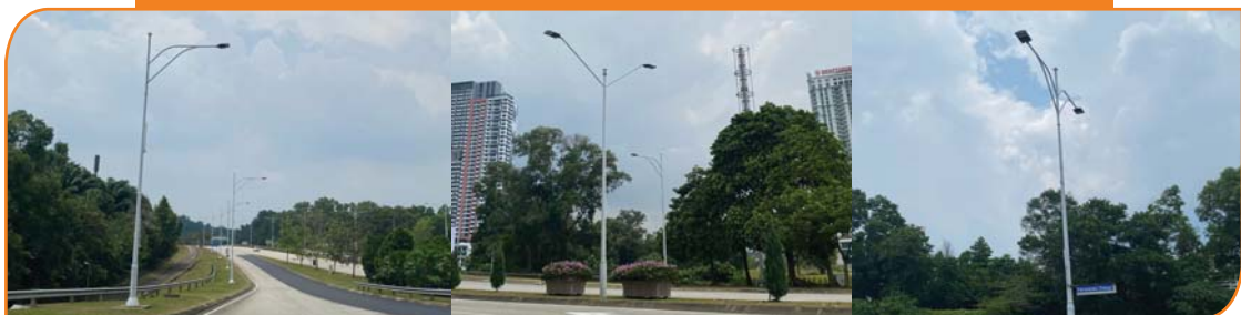
OLE Dura ST at Putrajaya, Malaysia
